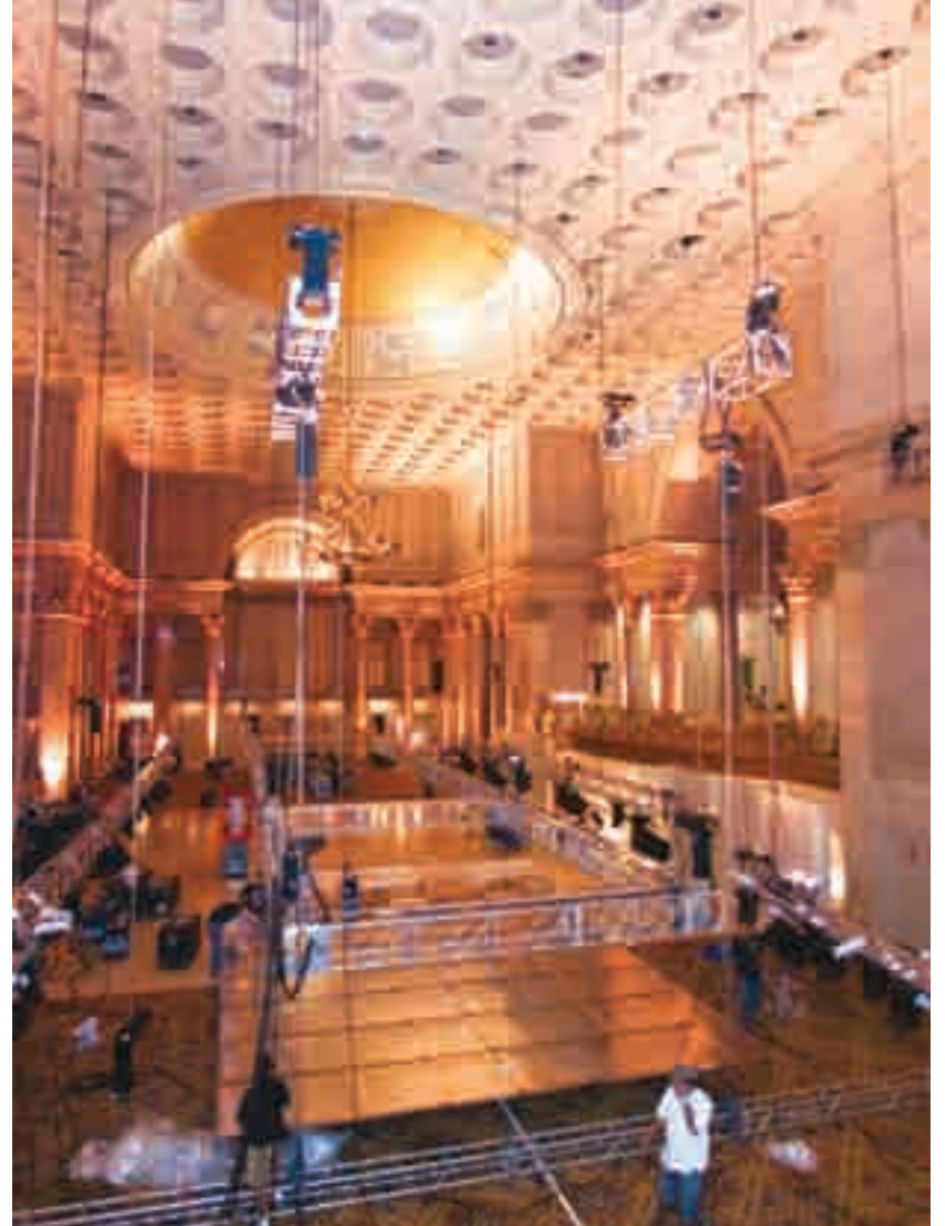
FRIDAY The priority on the first official day of installation was to rig all trusses and the reflective ceiling. OBO connected 31 four- by 23-foot mirrored panels on-site and hung them using an elaborate system of metal linking devices that enabled the team to level them.
