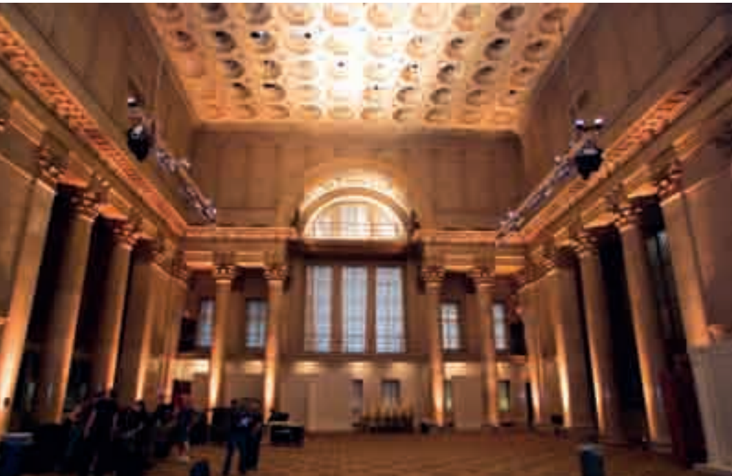
FRIDAY The priority on the first official day of installation was to rig all trusses and the reflective ceiling. OBO connected 31 four- by 23-foot mirrored panels on-site and hung them using an elaborate system of metal linking devices that enabled the team to level them.
