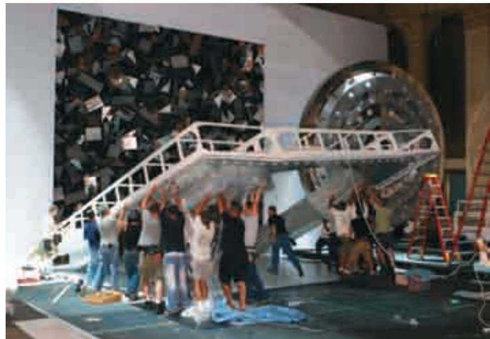
FRIDAY The priority on the first official day of installation was to rig all trusses and the reflective ceiling. OBO connected 31 four- by 23-foot mirrored panels on-site and hung them using an elaborate system of metal linking devices that enabled the team to level them.
